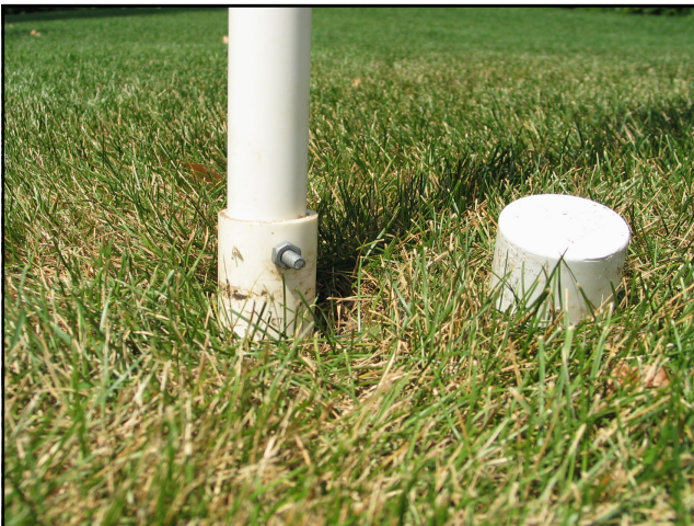
Slip the post in the mounting pipe and then insert the mounting bolt through the post and mounting pipe.
