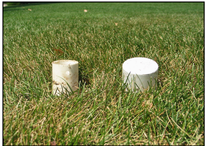
To install the sign post, remove the cap and pull up the pipe a few inches.
